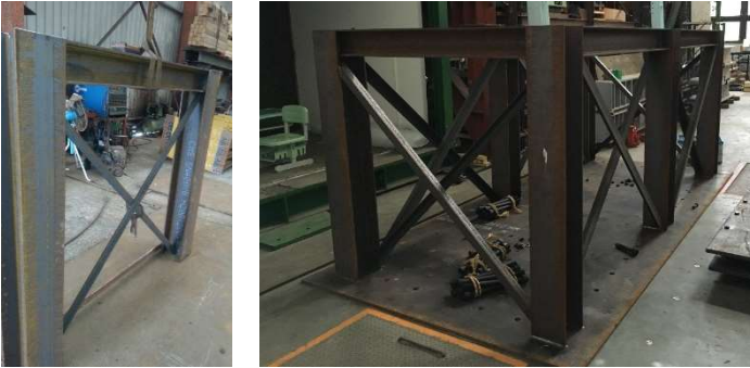
Construction of superstructure
