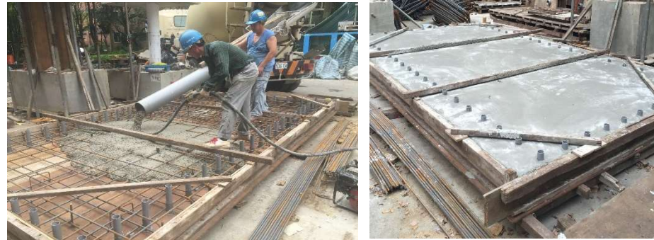
Casting of concrete layers
