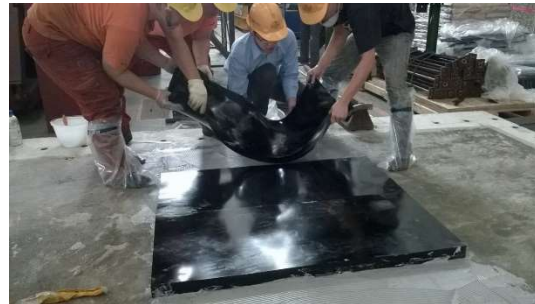
Construction of 1D periodic foundation
